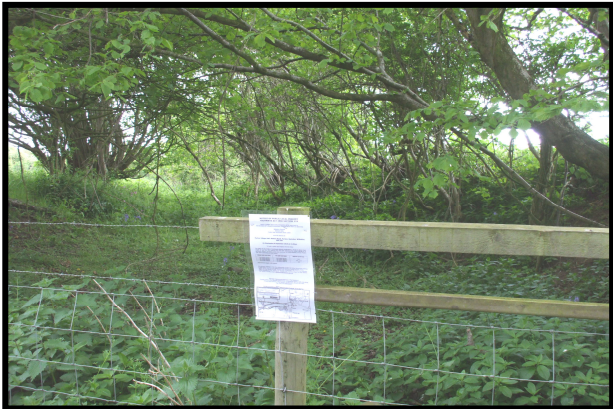
Existing route at points B (2010)
