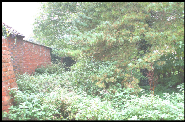
Existing route near point A (2007)
